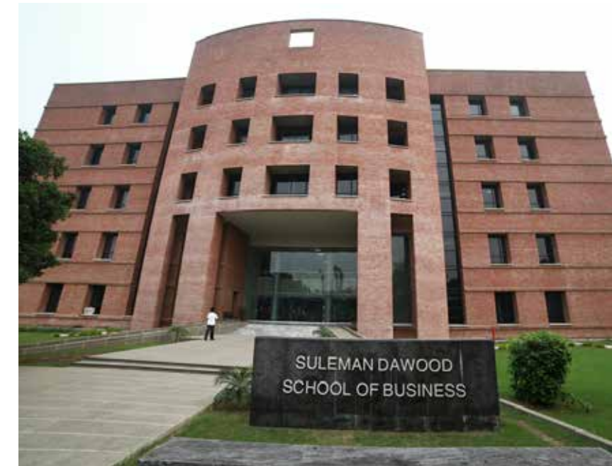
A front view of Suleman Dawood School of Business
